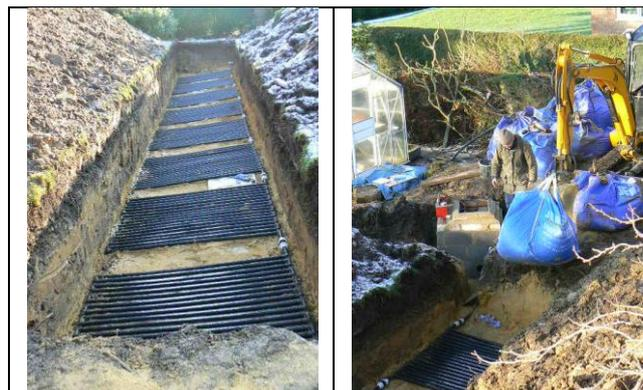
Pictures show the ground source heat pump pipes, backfilling and the manifold.
